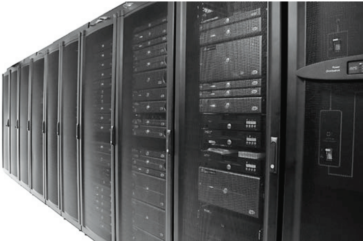
Racks of web servers
